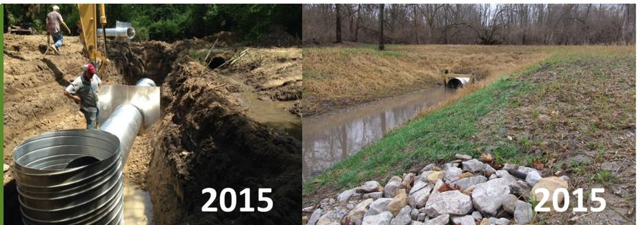
This drainage and erosion control project along a trail at Sand Creek Conservation Area was completed in 2015. It improves water quality, prevents soil erosion, and dangerous trail conditions by slowing the flow of water. As a result, less sediment washes into Lake Decatur, keeping our drinking water cleaner for wildlife and area residents.
